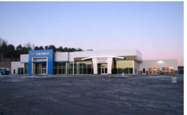
This building includes a geothermal climate control system. 18 holes were dug 360 feet below the dealership, with the purpose of consolidating heat from ground water to heat the building or redistributes heat into groundwater when cooling. This project also includes additional office space, a new retail showroom, and maintenance facility for both incoming, and outgoing vehicles.
